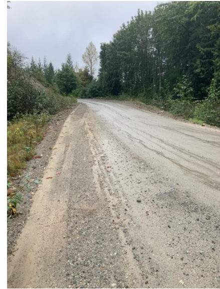
Approach from Left Bank when facing downstream
